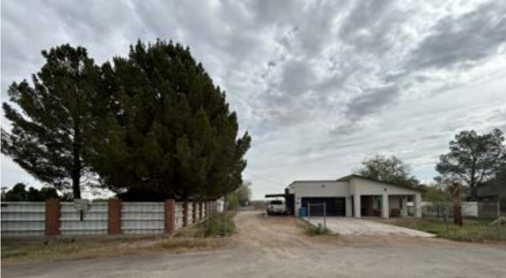
View of the property from F. E. Jackson Rd.
