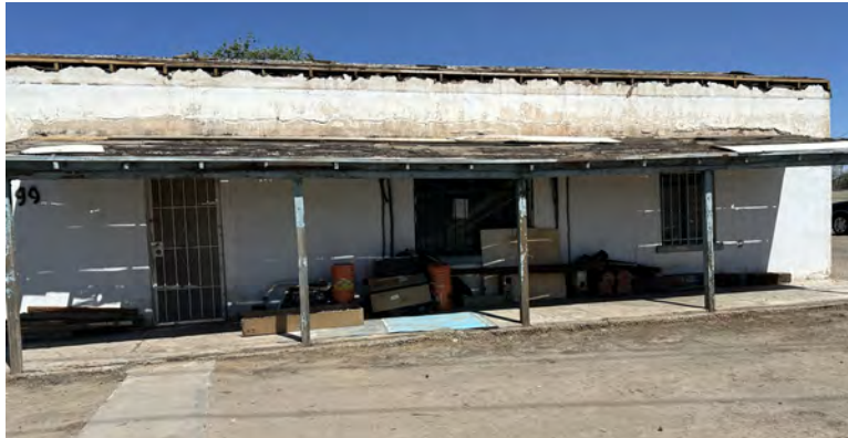
View of the property from Socorro Rd.
