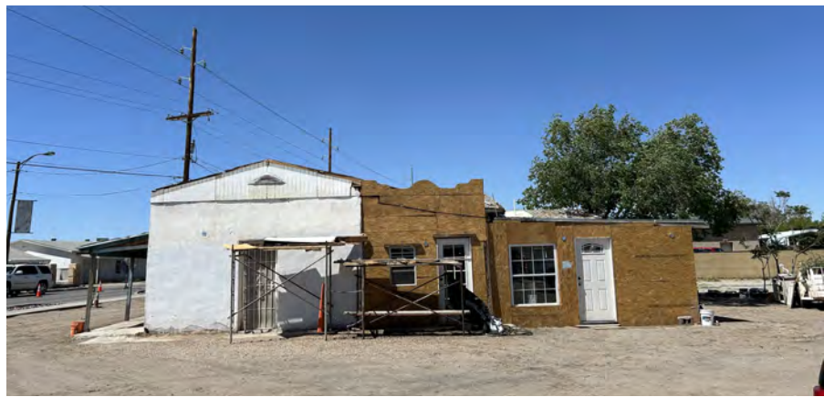
View of the property's right side from Buford Rd.
