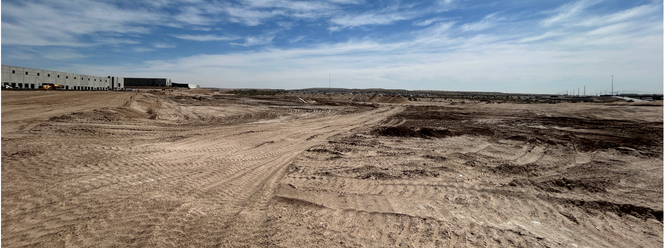
View of Gateway Industrial Unit Two
