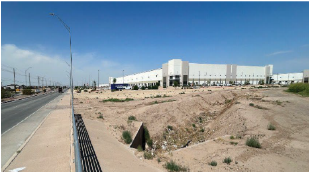
View of property from Nuevo Hueco Tanks
