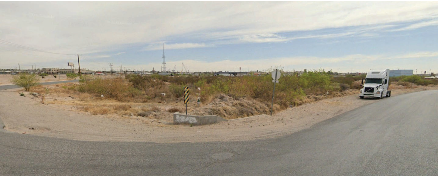
View of property from corner of Alyssa Rd and Stockyard Dr.
